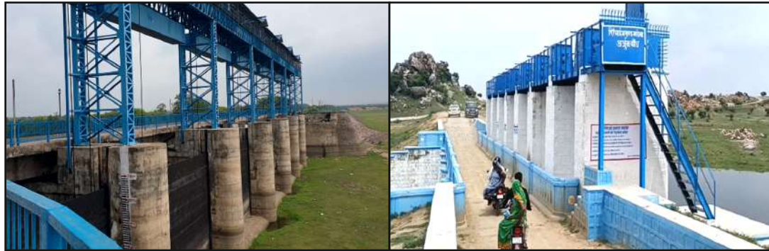
(a) Arjun Dam
